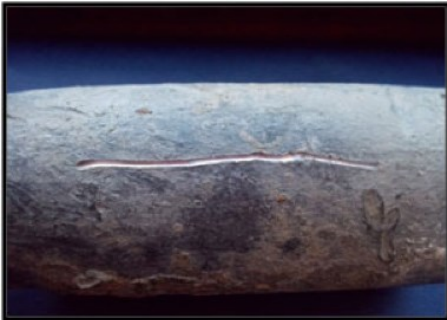
Key scratch on lead pipe. (photo courtesy of US EPA Region 5)
