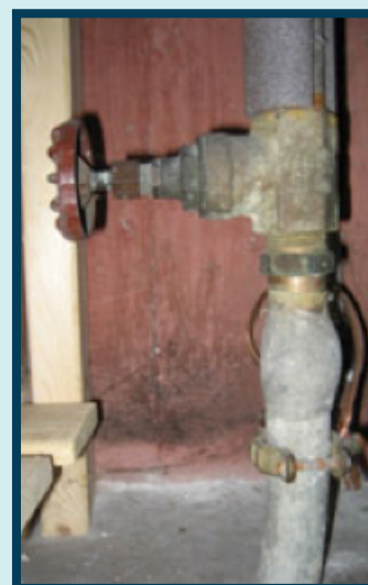
Lead service lines often have a "bulb" shaped connection. (photo courtesy of US EPA Region 5)
